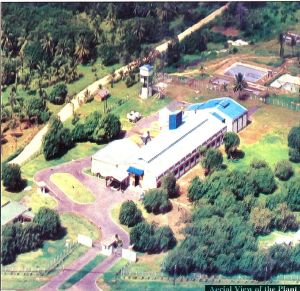
Aerial View of the Plant
