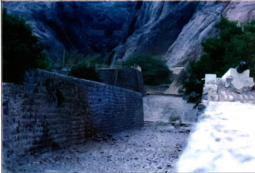
Jabal Huqqat: Sheikh Al-Ahmar has new construction going on there
