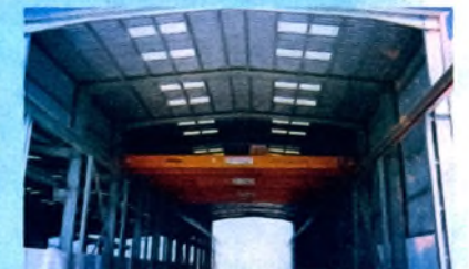
Stores and Workshop, NPCC, Abu Dhabi, UAE
