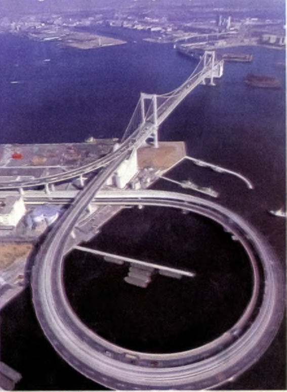
Rainbow Bridge, one of the famous bridges on the Gulf of Tokyo
