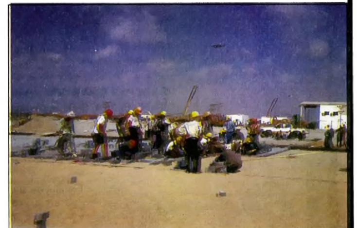
While paving of the Terminal Container Road.
