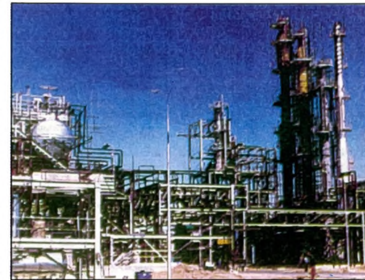
Isfahan Coal Tar Refinery
