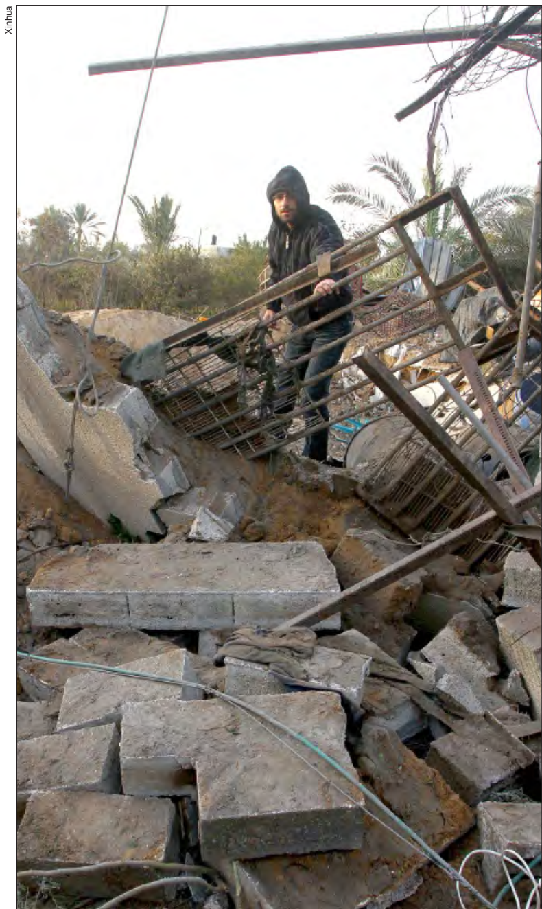
GAZA, March 6, 2011 — Palestinians survey the damage at the Islamic University building after Israeli air raid overnight, in Gaza City on March 6, 2011. Israeli warplanes struck with missiles on Saturday night several targets in the Gaza Strip in response to earlier homemade rockets attacks launched by Palestinian fighters.
