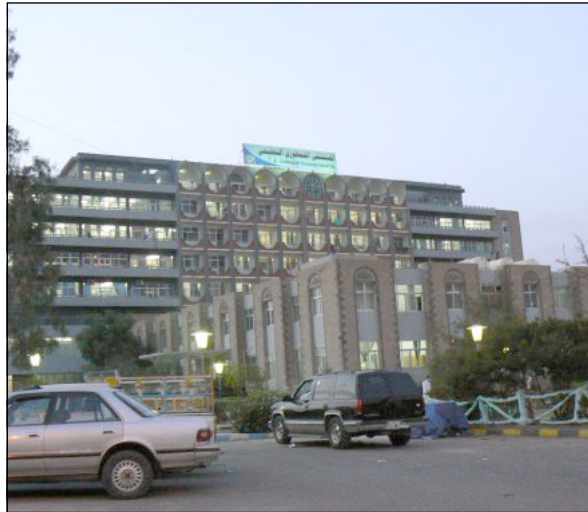
One of Yemen's largest hospital, Republic Hospital
