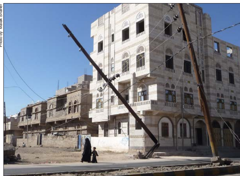
The electricity pole was hit in accident six months ago but has no power. However, residents say it could fall at any moment.
