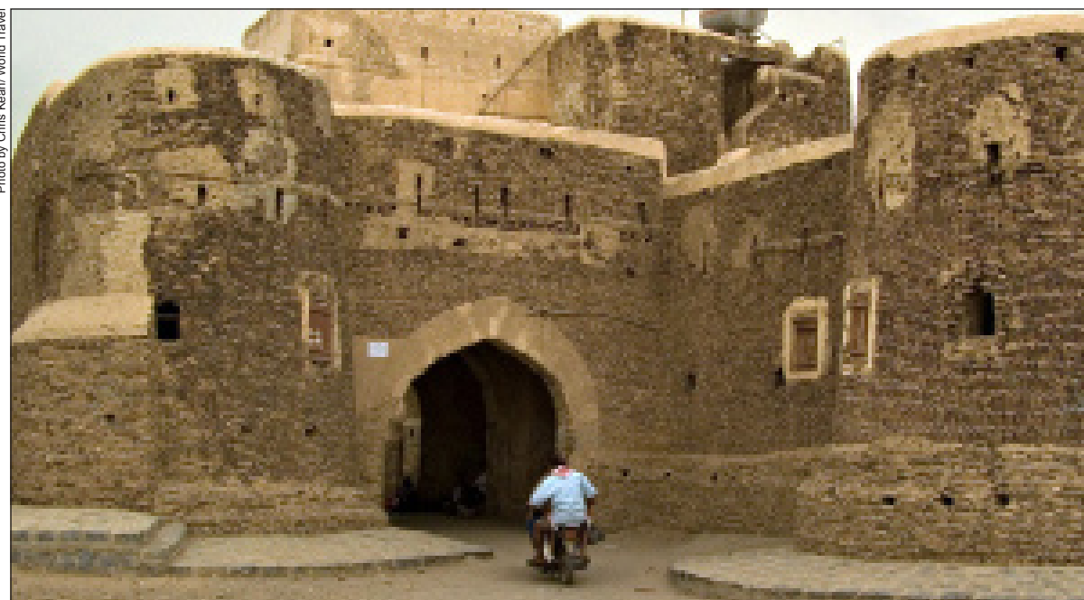
Old city gate in Zabid, which had seven historical gates surrounding the old city. Only four remained until today.
