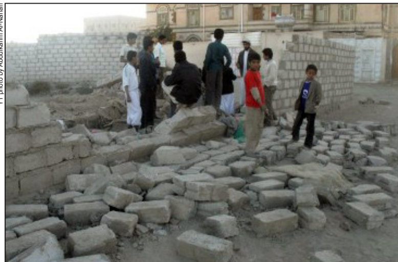
Part of the house where the explosion occurred in Dhamar.
