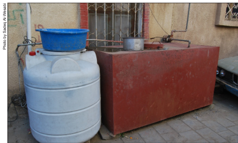
Fiberglass tanks are the best replacement for unhealthy iron water tanks, according to Dr. Rami Al-Maqtari.
