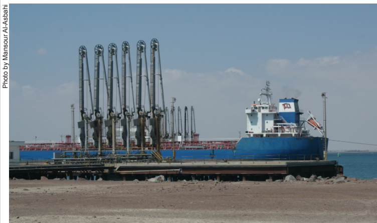
A committee of the General Authority of Maritime Affairs has been set up to investigate the sea contamination on the Yemeni water on Ras Al-Ara.
