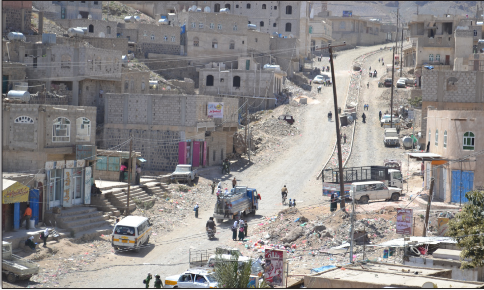
Al-Sonaina Road is rugged and dirty, but attempts to repair the road have been in vain.
