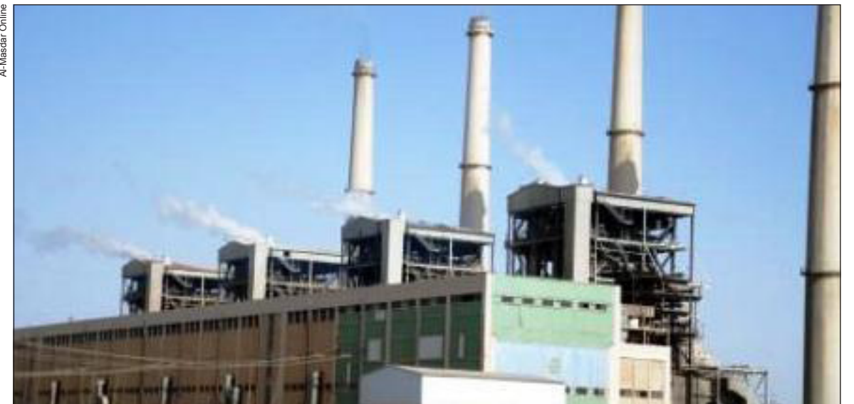
Marib power station is facing increasing threats from tribal bombs.
