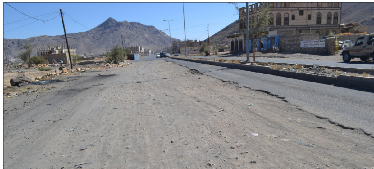
This is one of the many road projects across the country that was never finished. During the political instability of the revolution, laborers lost jobs as contractors struggled to continue.
