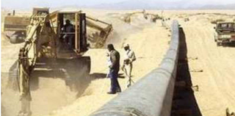
Workers fix the first oil pipeline blown up in 2013
