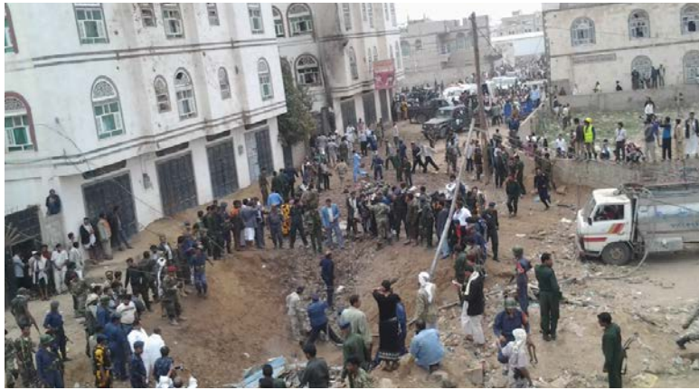
Three houses were damaged when the plane tore into this residential neighborhood.
