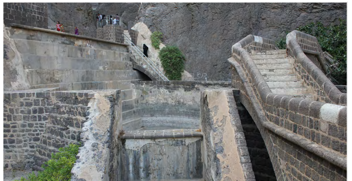
Rocks from Shamsan Mountain were used to build the walls of the cisterns.
