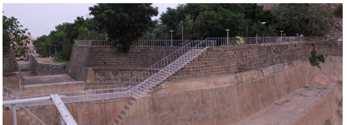
The cisterns originally had a combined capacity of about 20 million gallons, according to one estimate.
