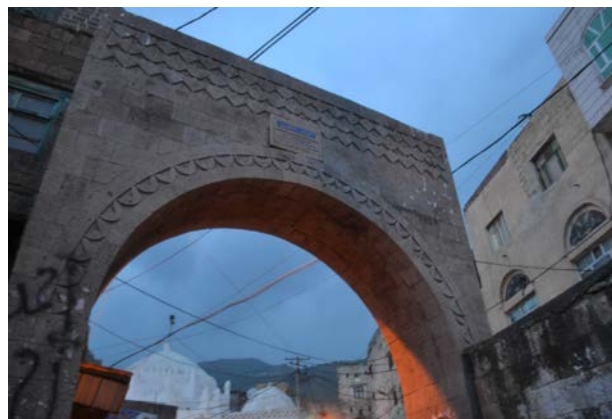
One of the city's entrances after renovation.
