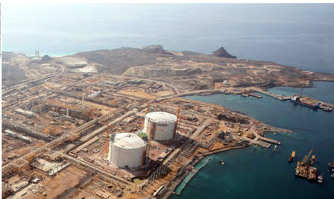
Balhaf Terminal exports up to 12.5 billion cubic meters of gas per year.
