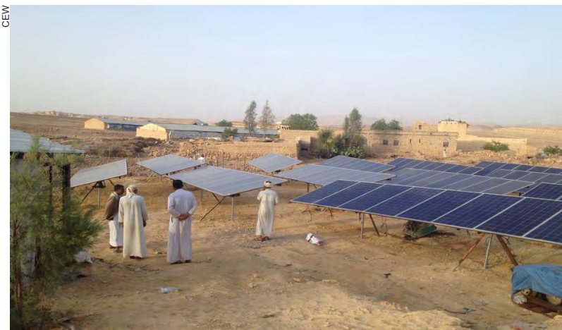
Visitors come every day to see in person how the solar pump system pumps water for agricultural irrigation.
