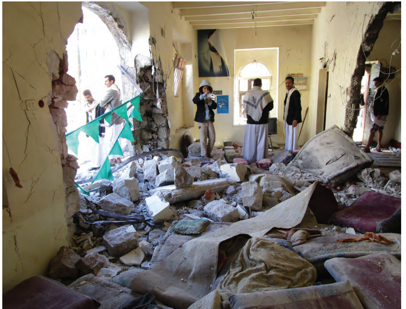
The first floor of Naji Mahi Al-Deen's home in Sana'a's Salah Al-Deen neighborhood following an IED explosion that took place Sunday morning.
