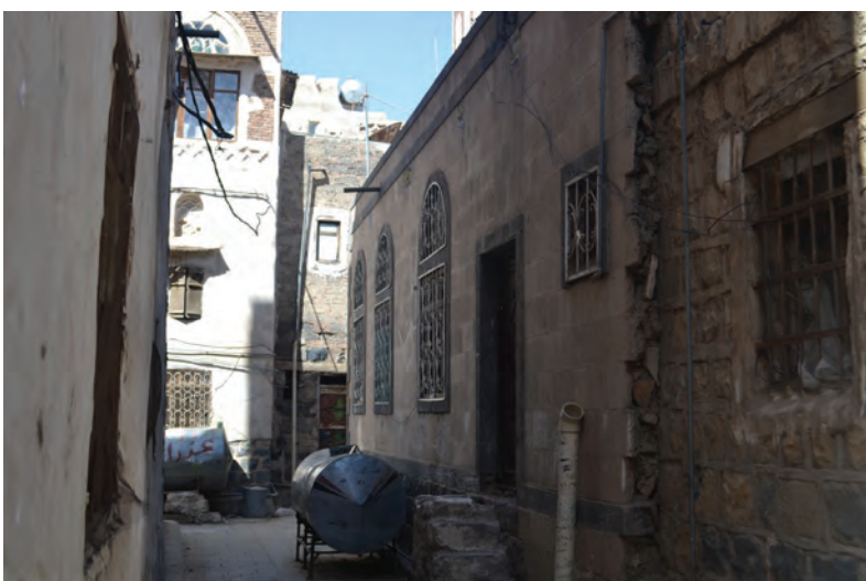
Home in Sana'a's Old City built in violation of the neighborhood's traditional architectural style.
