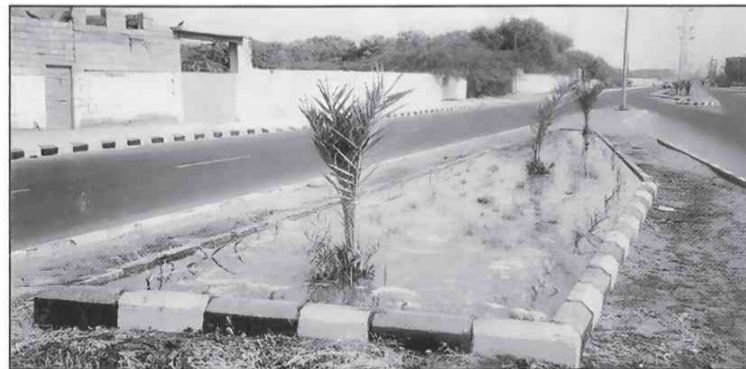
Renovation complete in Duraimi St.
