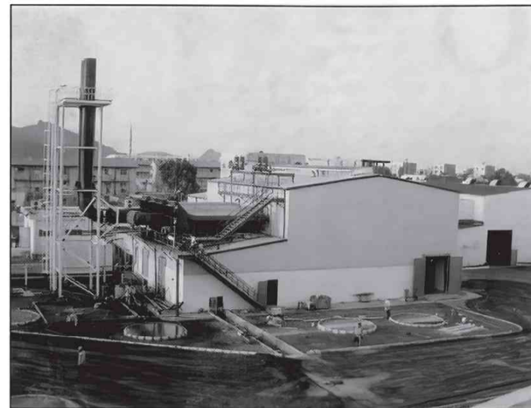
Aden electricity station
