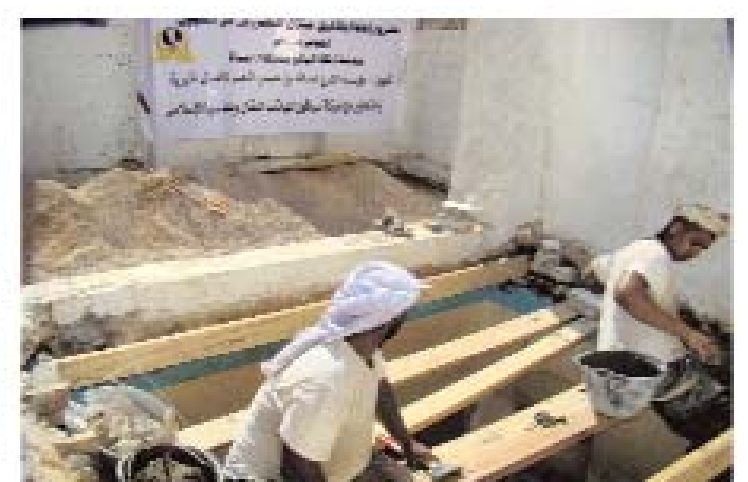
Renovations in progress for damaged houses
