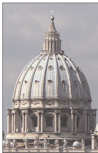
The dome of San Pietro in Vaticano (Saint Peter's Basilica) in Rome, seen from the roof of Engelsburg.
