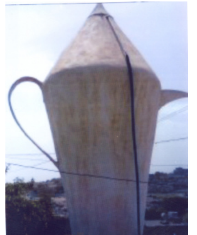
Water tank made of fibercement and iron.
