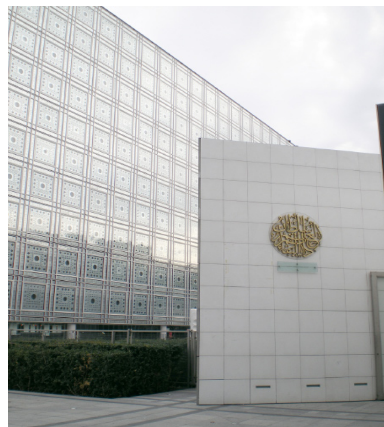
The main entrance to the Institute of the Arab World through the facade composed of numerous mashrabiya squares.
