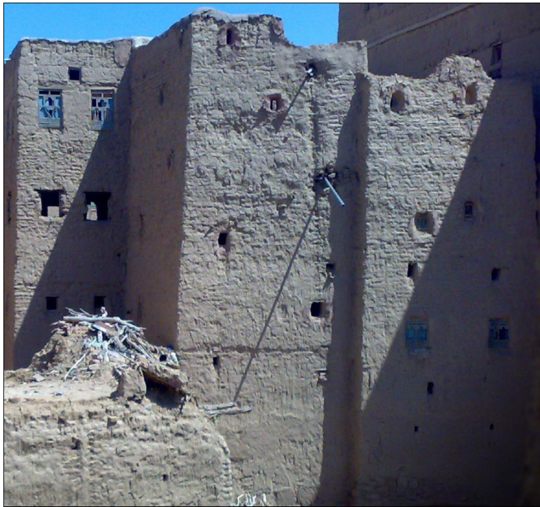
An old 200-year earthen house with cow dung remains applied around the windows.
