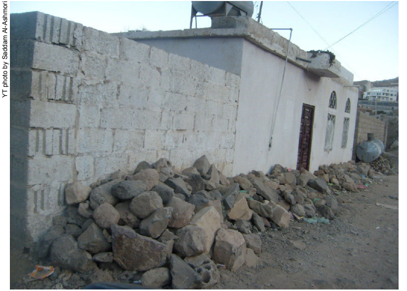
With no modern drainage system in the area, residents in Al-Ashash have piled stones outside their houses to protect them against possible floods.
