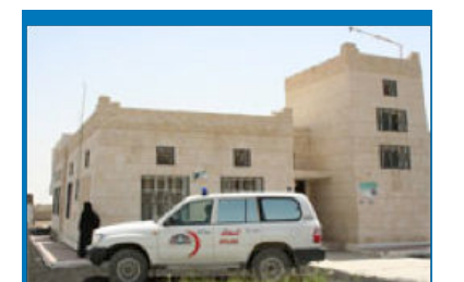
To provide doctors, nurses and other skilled medical workers with safe and healthy accommodation in a remote hospital in Yemen's Marib Governorate, U.S. aid has built housing and supplied an ambulance to transport critical patients.
