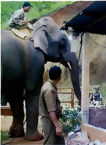
Elephant demolishes an illegally built house in a protected forest area around Guwahati, India. REUTERS/Utpal Baruah
