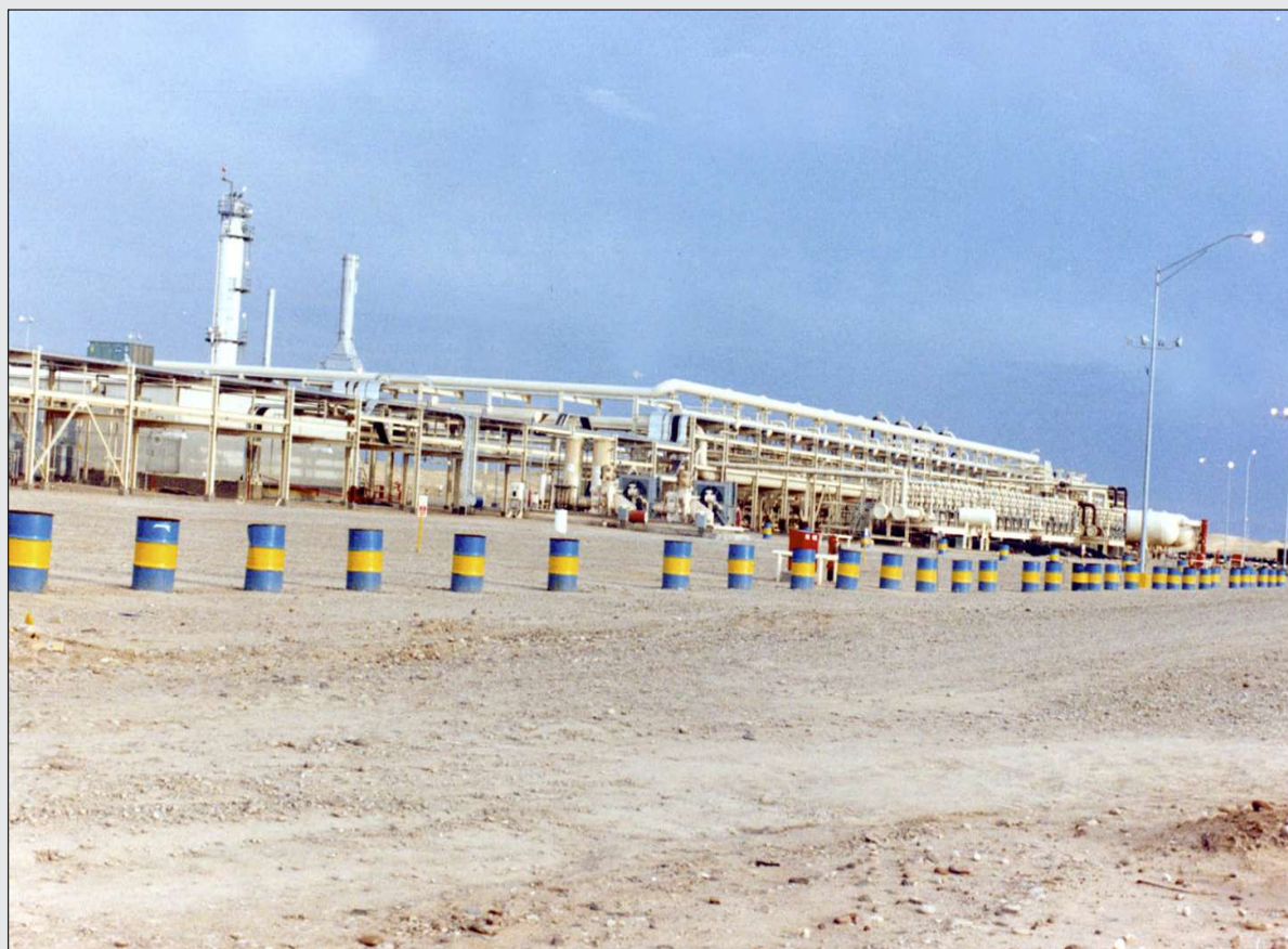
Natural gas refinery in Yemen.
