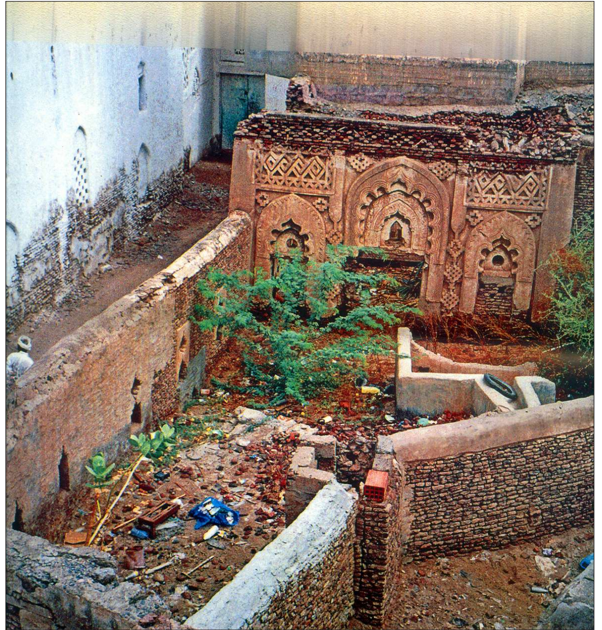
The remains of a wonderfully built piece of art juxtaposed by side garbage in its yard. This should prompt the concerned people to act.
