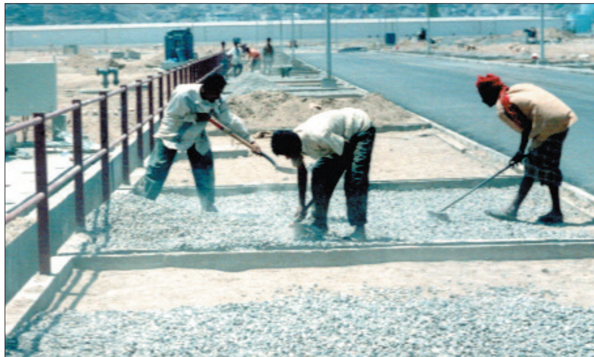
Workers performing street cleaning and paving works.
