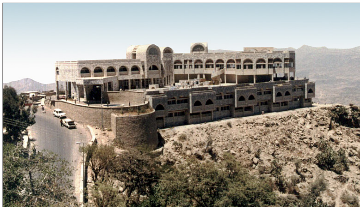
Sheikh Zayed Park.
