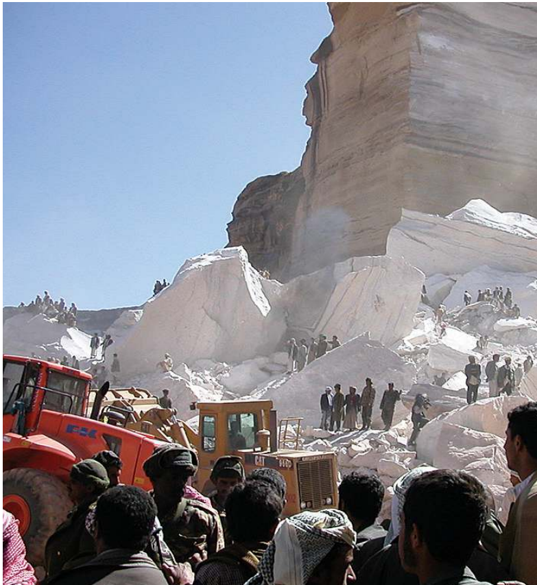
Rubble-removing operations done by heavy machinery.
