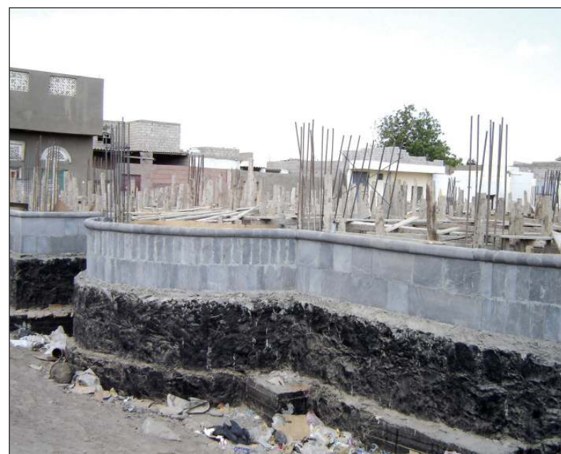
Post office being constructed in Dar Sa'ad
