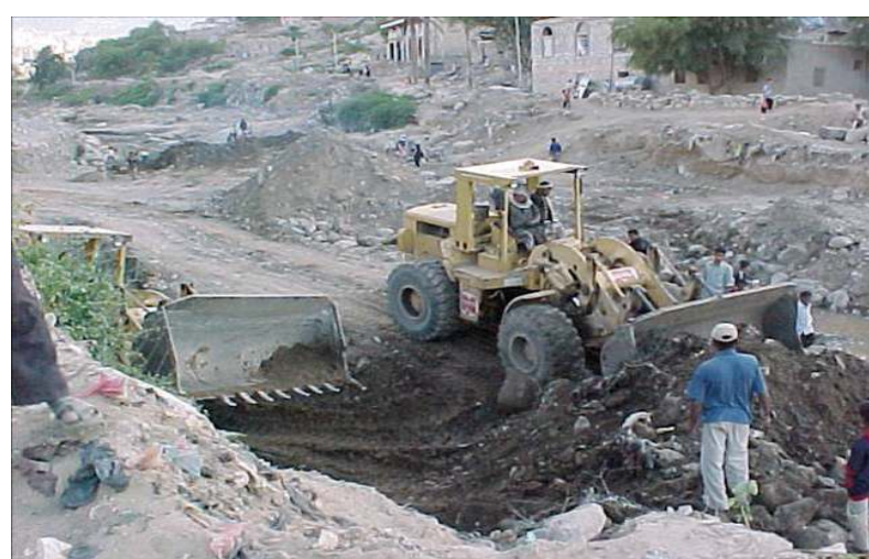
Flattening Wadies to build Gabions
