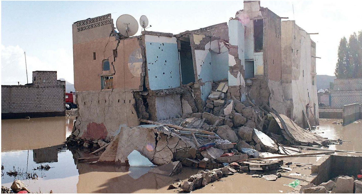
One of the houses damaged by the flood.
