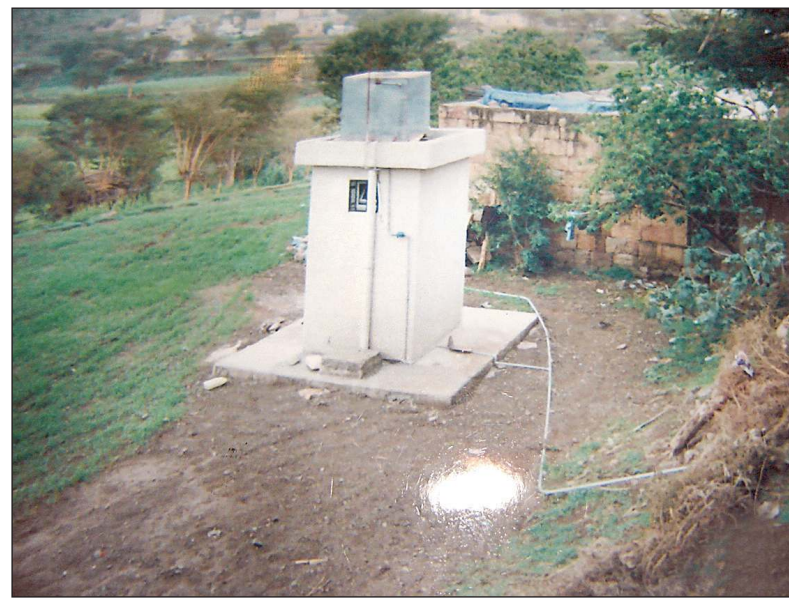
View of water and sewage project in Ibb.
