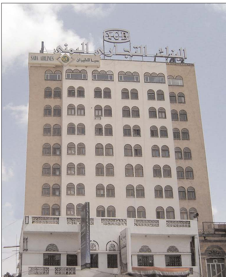
Yemen Commercial Bank (YCB) headquarters
