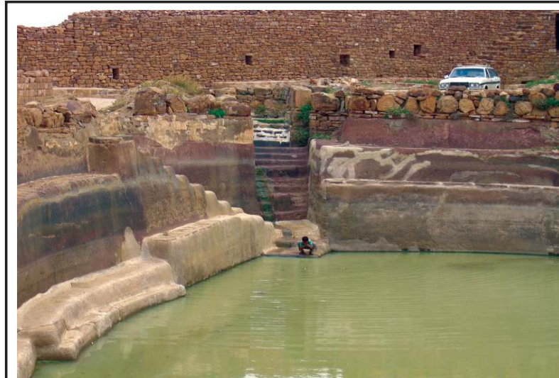
Jadaan Cistern before rehabilitation.
