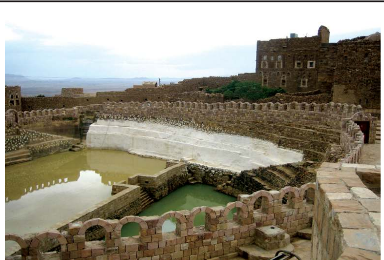
Jadaan Cistern after rehabilitation.
