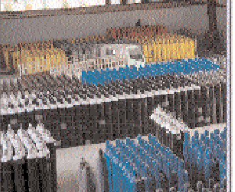
Oxygen storage facility
