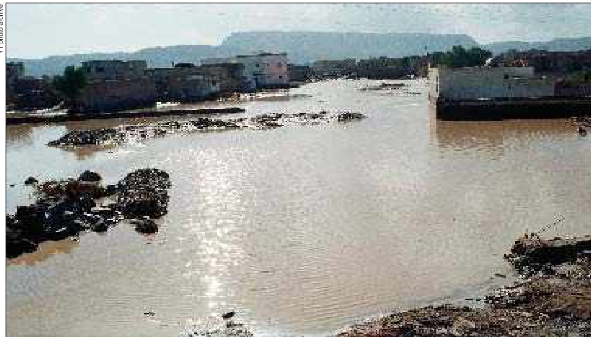
Flood in Taiz governorate causing damage to the infrastructure and land in 2006. Flooding occurs during the monsoon season, leading to a loss of productive agricultural lands along the wadis, increasing sedimentation and significant widening of the downstream wadi bed.
