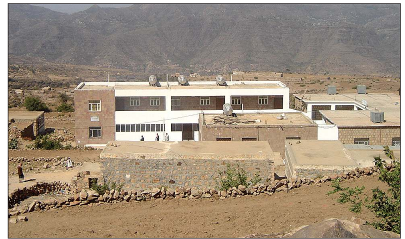
A view of Al-Thawra Medical Center in Al-Selu district which has been expanded and equipped by USAID and US Defense Civil Affairs Section.
