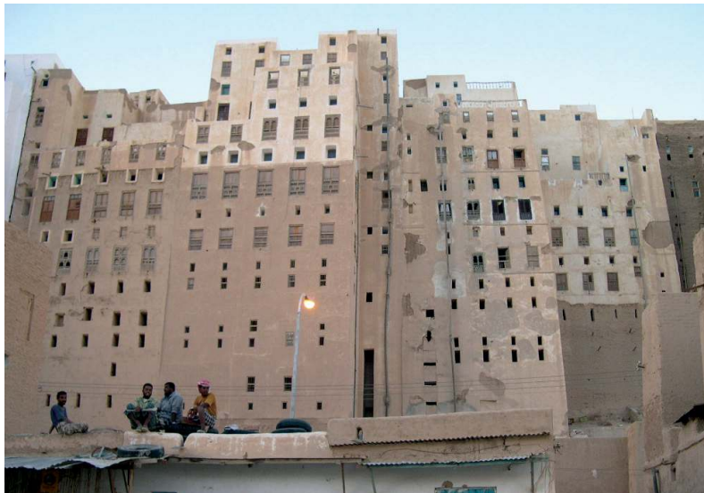
The Shibam Urban Development Project has approached the city as a living community rather than a historical artifact frozen in time.
