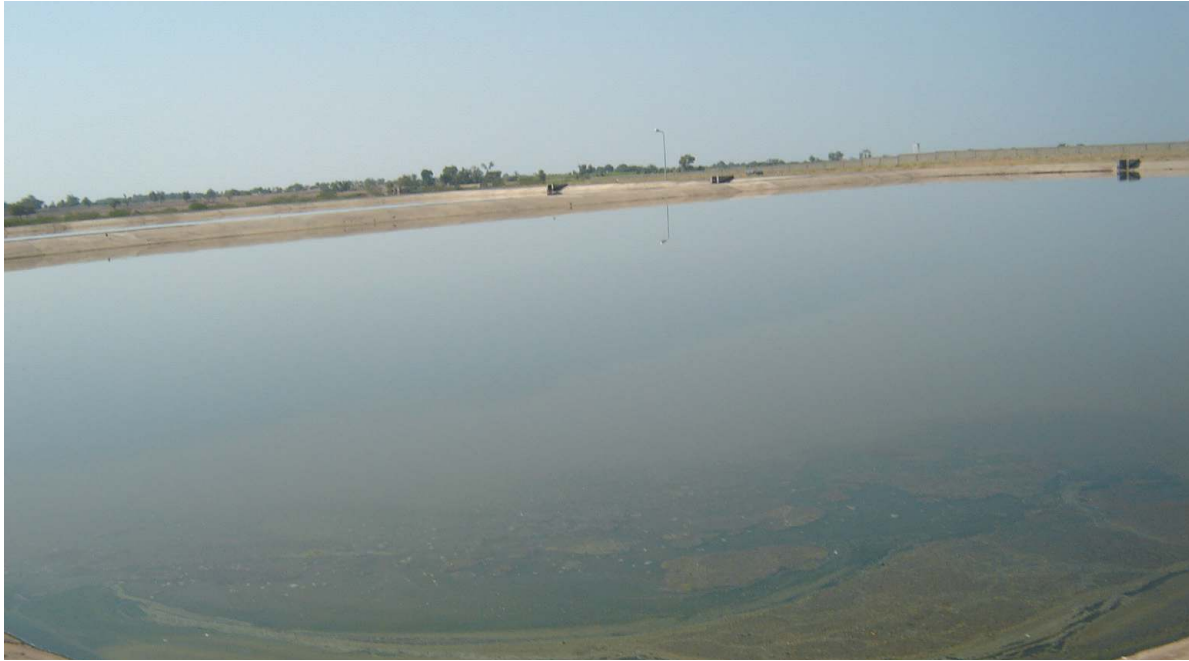
Water supply and sanitation project in Bait Al-Faqih.
