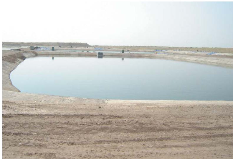
Water supply and sanitation project in Zabid.
