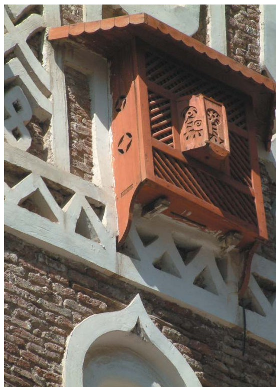
Decoration is one of the forms of beauty within the Old City of Sana'a and is found on nearly all of its buildings. Photo by Fadhl Al-Amdi
