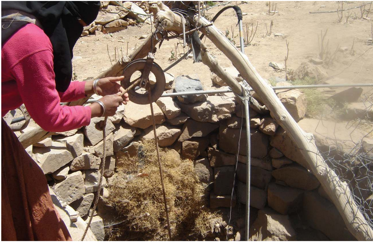
Out of 20 wells in the village, only two still provide people with drinking water
